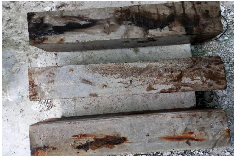
Figure : Beams after corrosion
