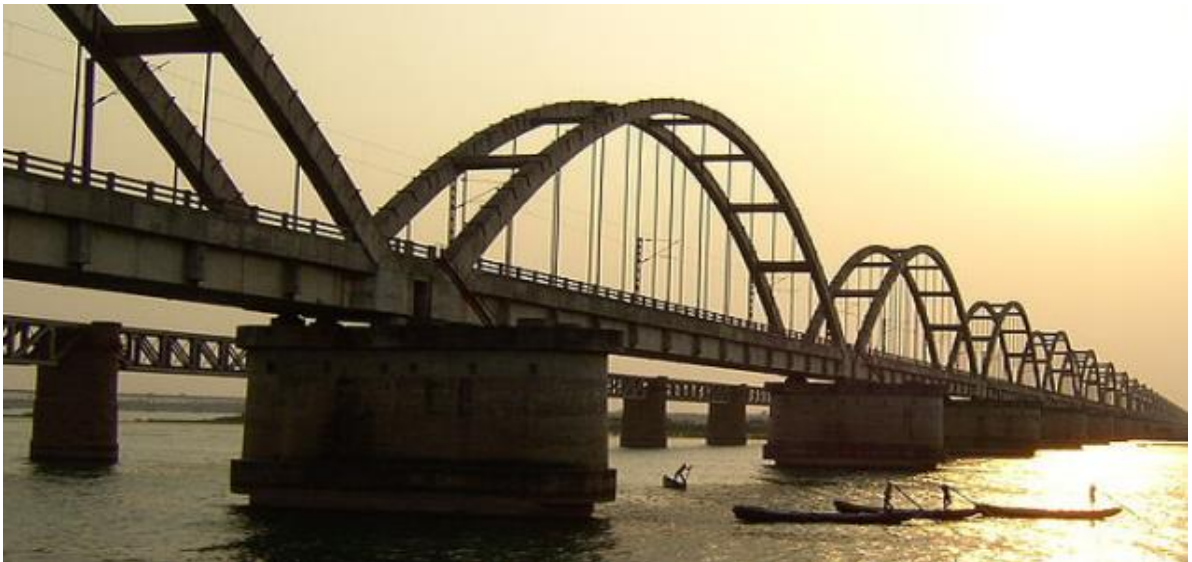
Fig. 1.3- Godavari Arch Bridge at Godavari River
