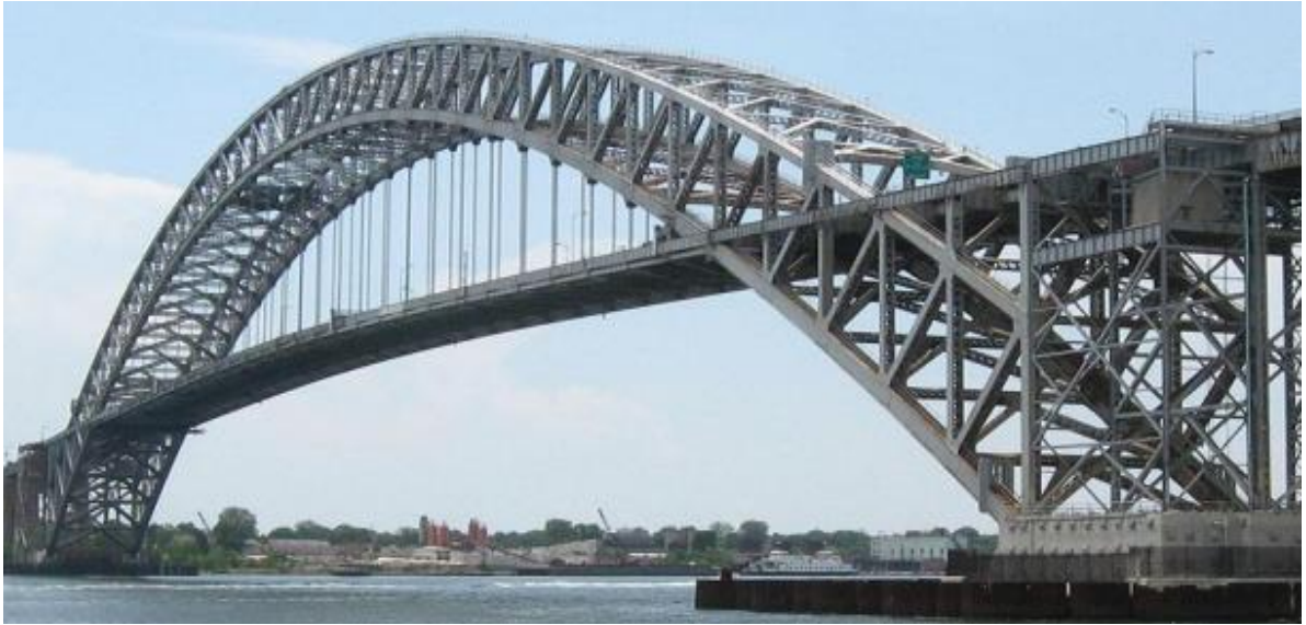
Fig. 1.2- The Bayonne Bridge, New York
