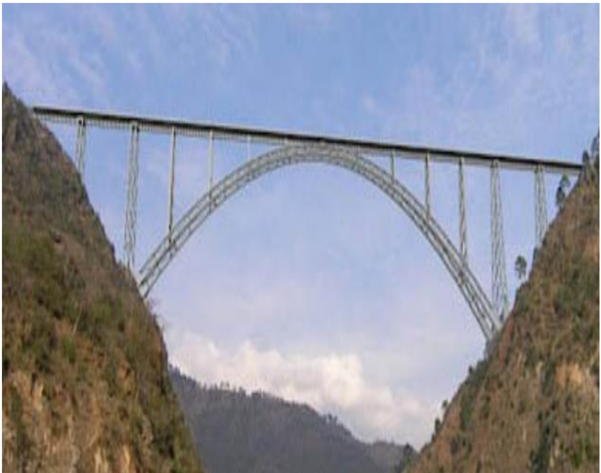
Fig. 1.1- Chenab Railway Bridge Katra, Jammu-Kashmir, India
