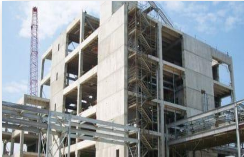
Fig. 1.1 Shear Wall in building (Source: www.theconstructor.org )
