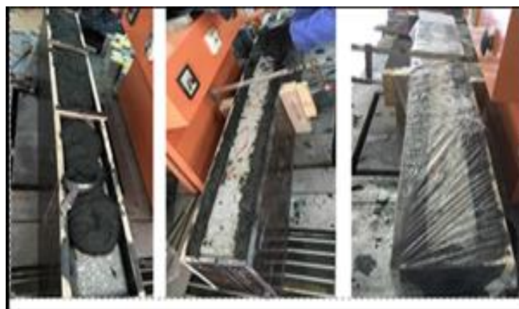
Fig. 3. Strengthening process using Sandblasting and UHPFRC in-situ Reinforcement Techniques
