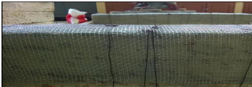
Fig. 5. Wrapping of Wire Mesh(U-Wrap)
