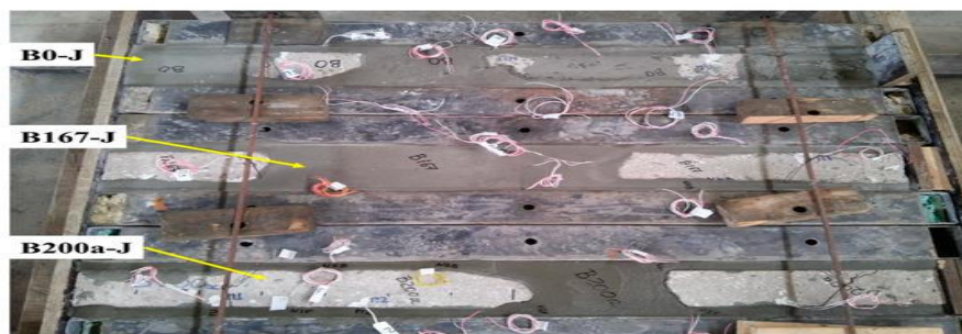
Fig. 1. Forming of U-Shaped Jackets with Gusting Cement Mortar Grout Matrix
