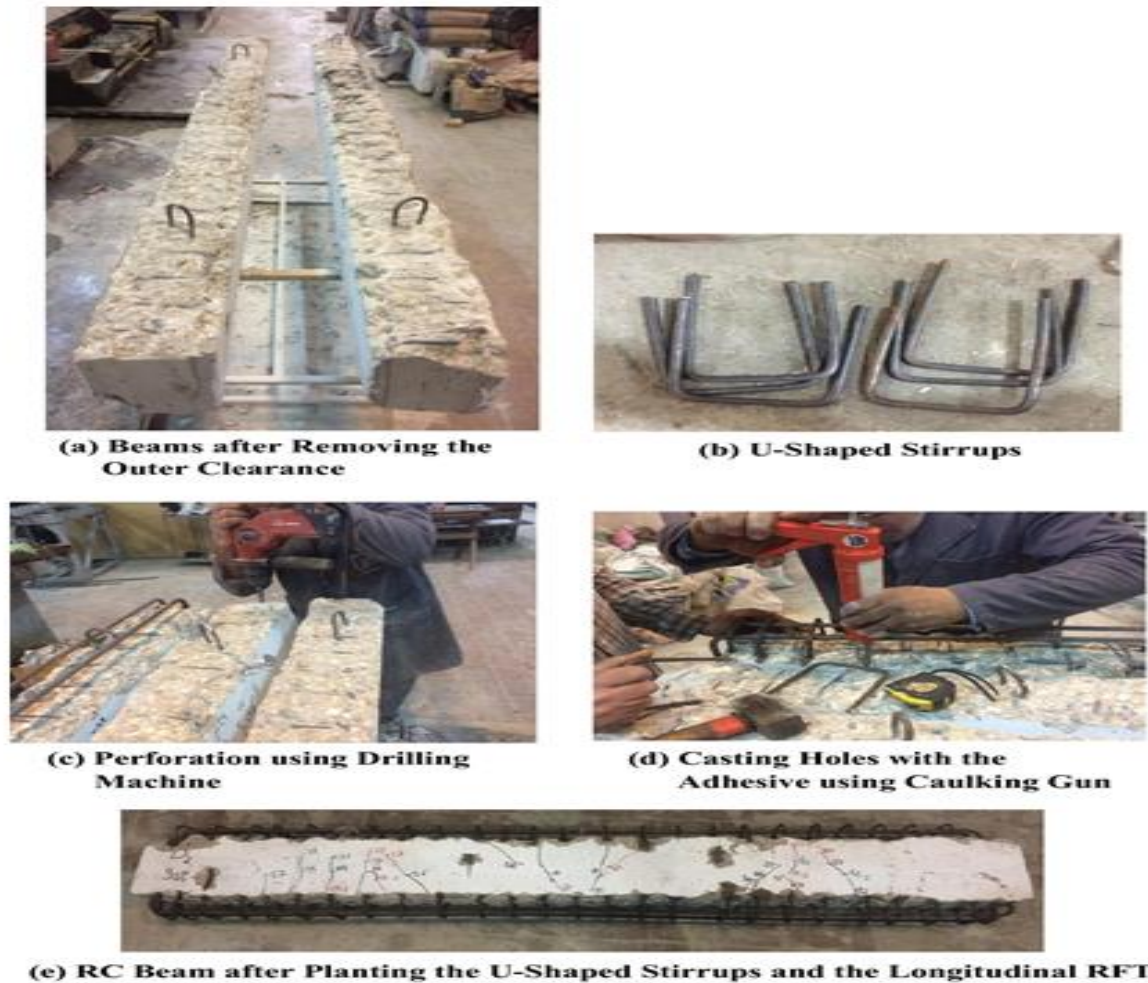
Fig. 2. Steps of Strengthening using RC-Layers
