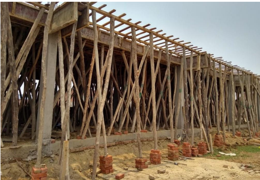
Fig.3.3-Formwork of a Building
