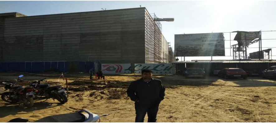
Fig.3.2- Levelling of Earth
