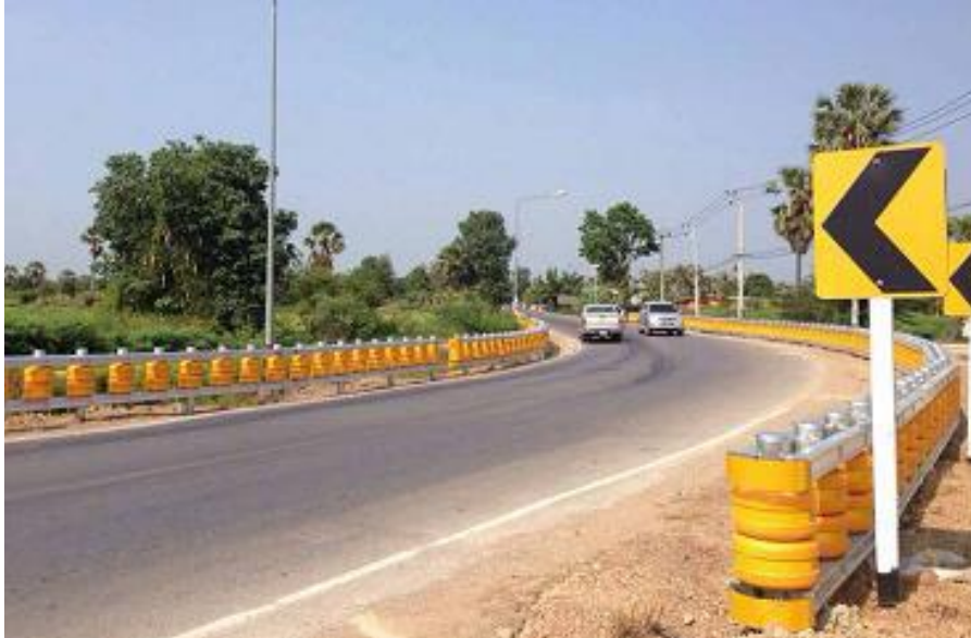
Fig. 1.14: Installation of barriers on existing barriers & new barrier construction
