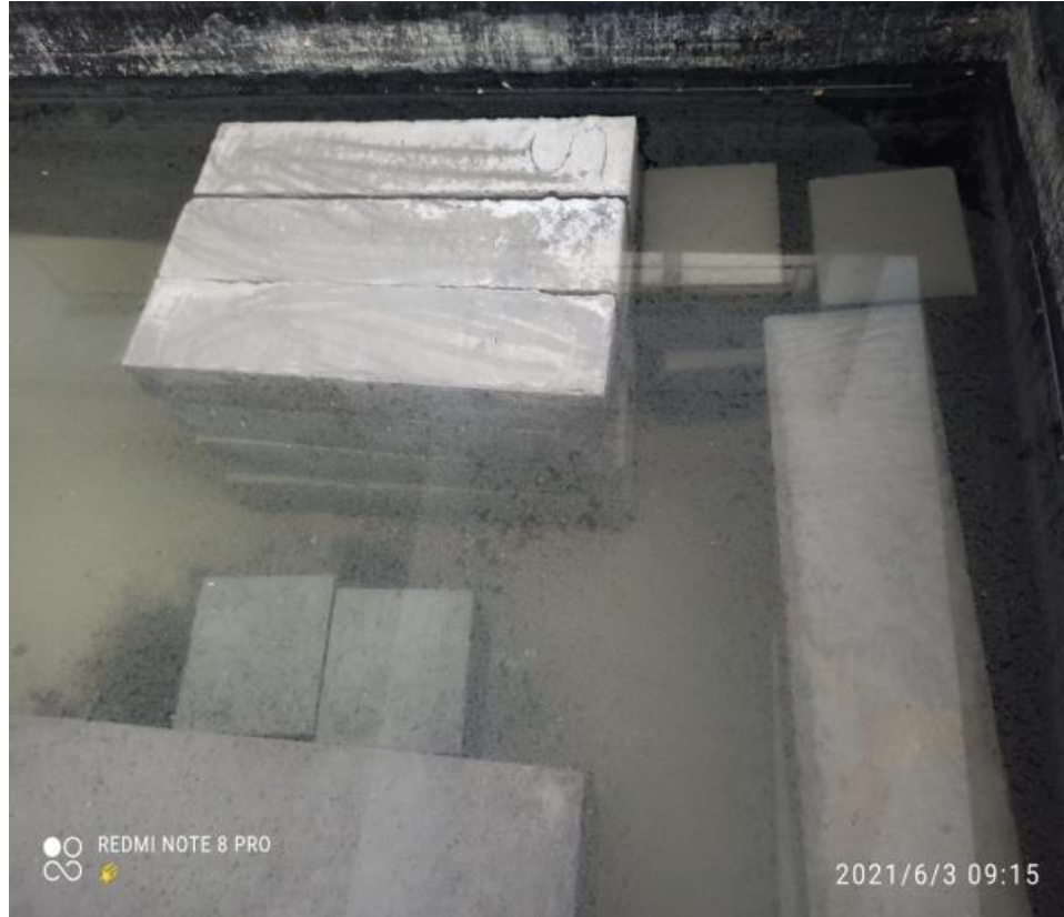
Fig3.3.3 curing of beam
