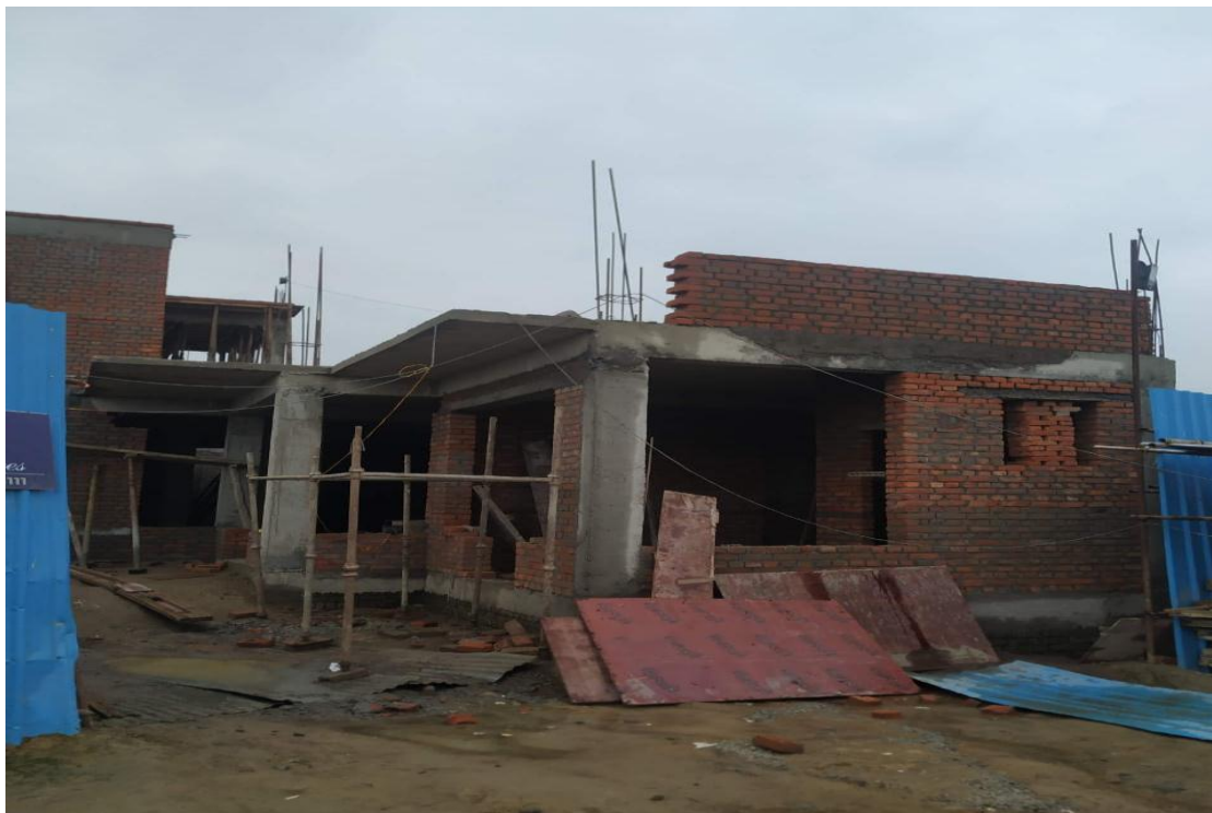
Fig 4.5: Brickwork and plastering
