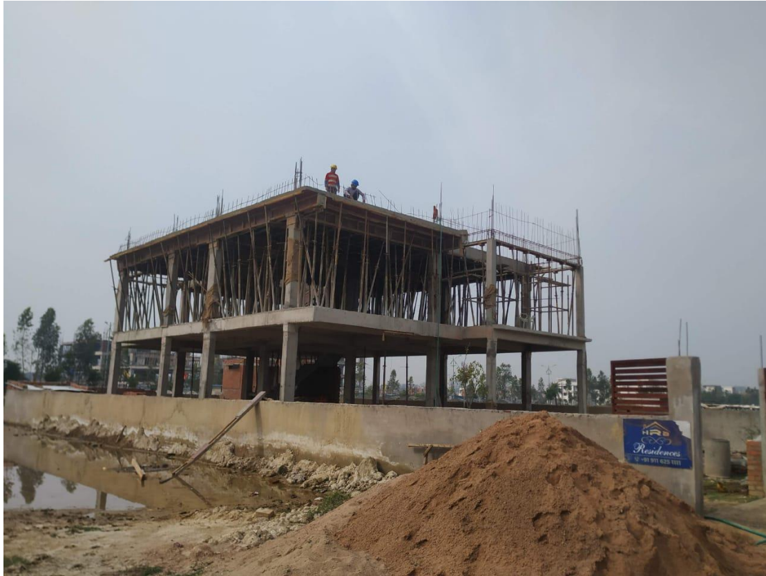
Fig 4.4: Form work and casting of slab
