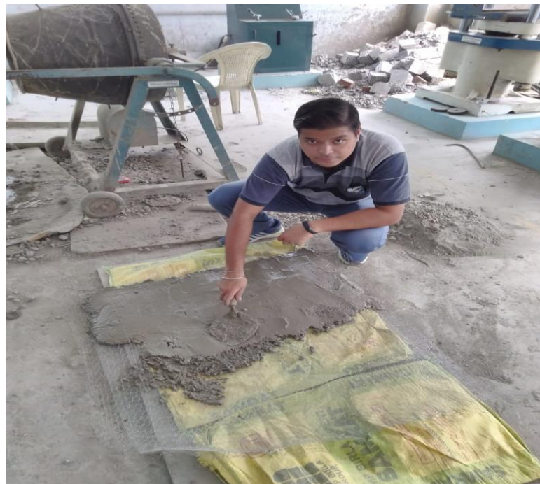
Plastering on wire mesh
