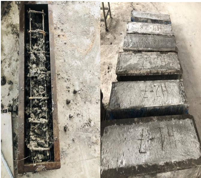
Fig 4.4 Casting of beams
