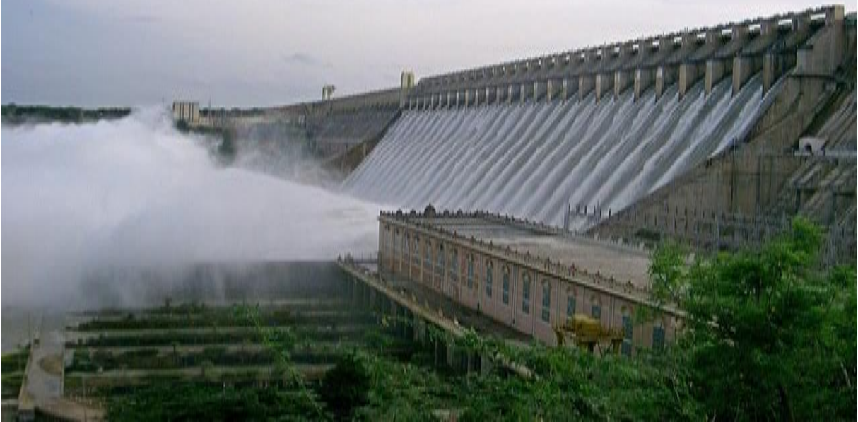
Fig 4.6 Nagarjuna Sagar Dam and the 810 MW pumped storage hydroelectric power plant on the Krishna River.
