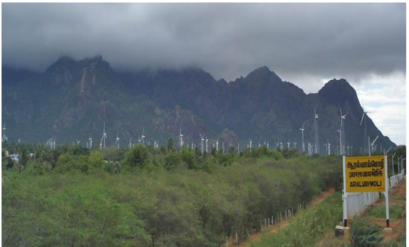
Fig 4.7 The largest wind farm of India in Muppandal, Tamil Nadu.
