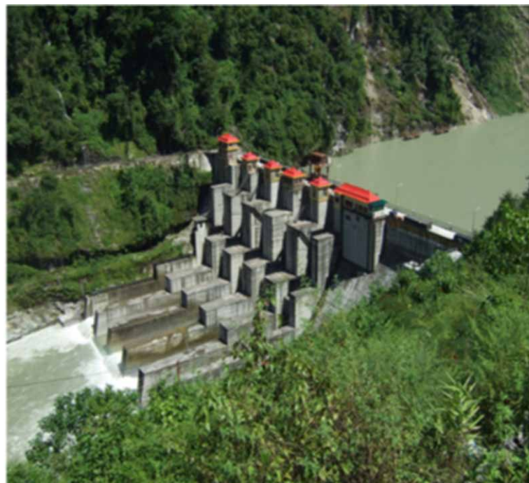
Figure 8. 510 MW Teesta-V power station in Sikkim (Iha, 2022)
