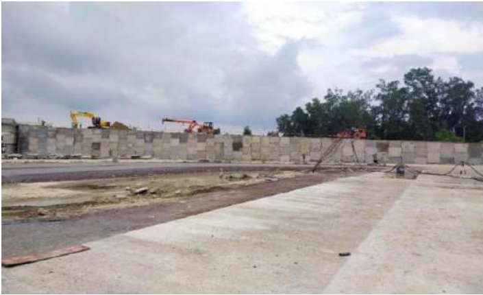
Fig 15: Precast RE Wall Panel erection
