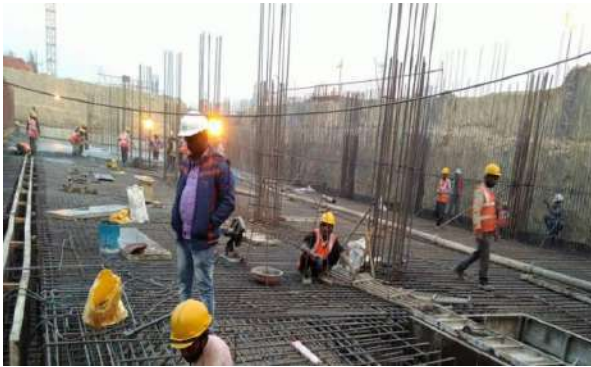
Fig 7: Raft foundation
