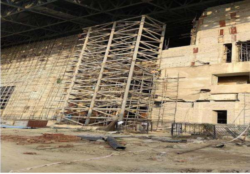
Fig 17: Lift Wall Tower
