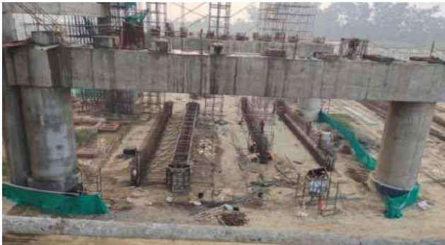
Fig 10: Pedestal above Pier Cap
