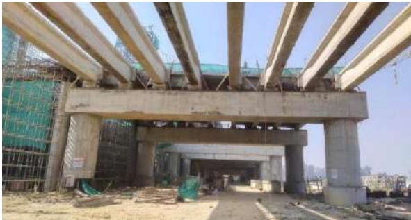
Fig 12: RCC Precast Girders Erection
