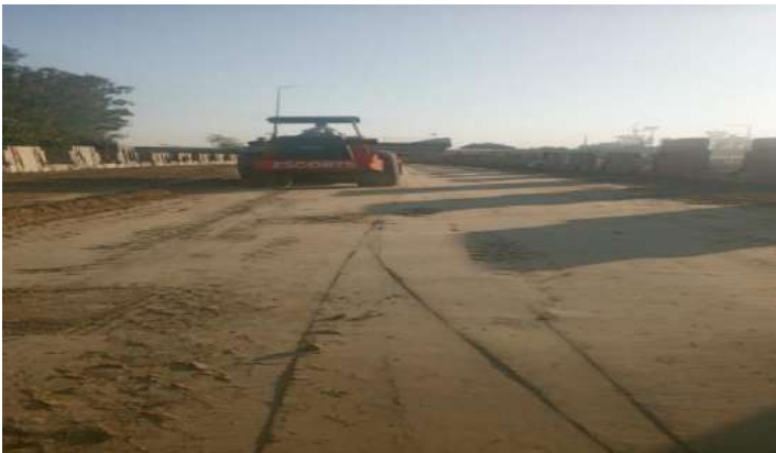
Fig 14: Soil Compaction work
