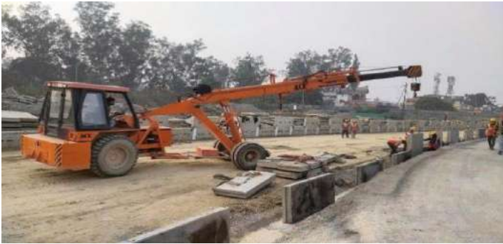
Fig 13: Precast RE Wall Panel erection
