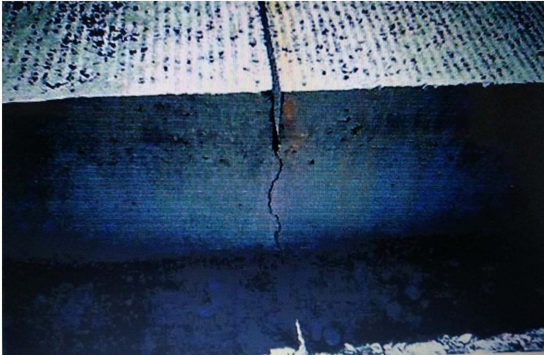
Fig 6.5.1 Aggregate Interlock
