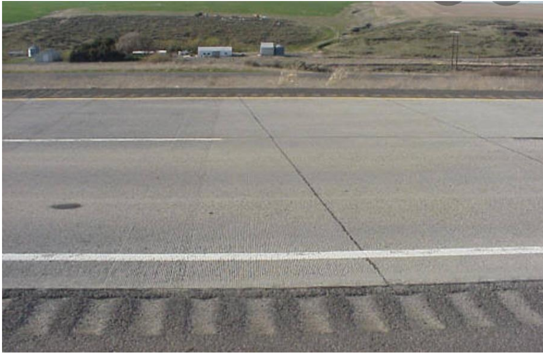
Fig6.3.3Skewed Contraction Joint
