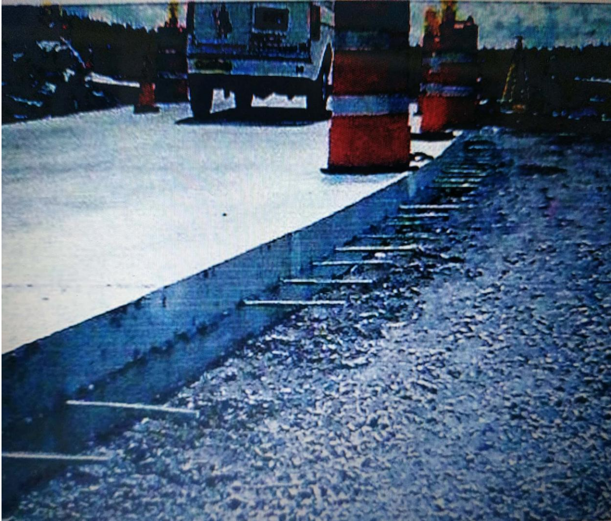
Fig6.8.1 Tie Bars along a Longitudinal Joint
