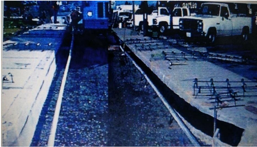
Fig 6.3.4 Roofing Paper Used For an Isolation Joint
